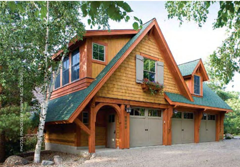
THIS PAGE: Murphy designed a clean, contemporary motor shop on the first floor with space for three cars, plus two 7,000 hydraulic lifts, a mechanical room with a built-in air compressor, and a separate snowmobile entrance with ski guides built into the floor.
